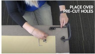
Align corner retainer bar with pre-installed plates.
